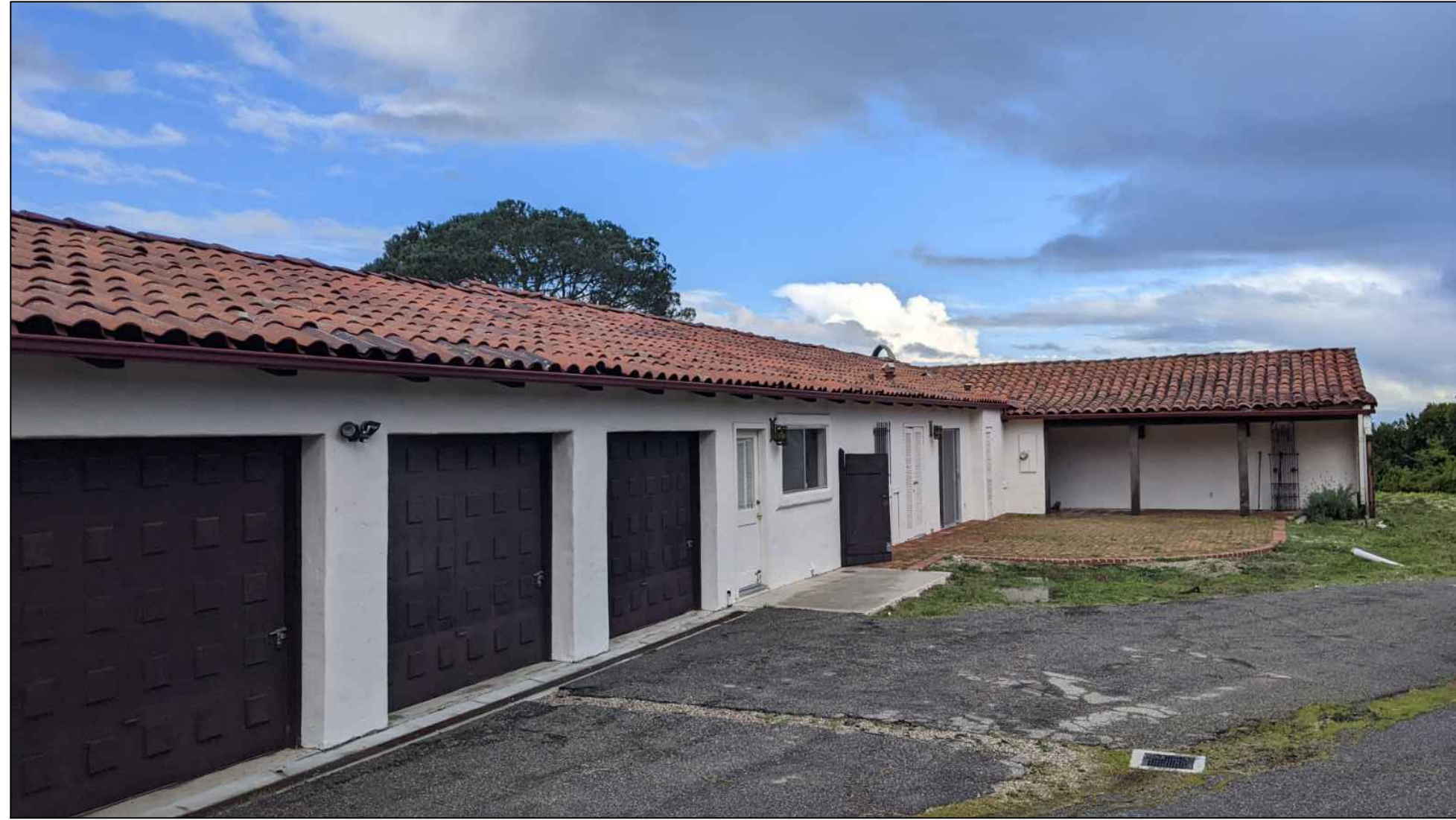
SOUTH SIDE EXISTING RESIDENCE TO BE DEMOLISHED
