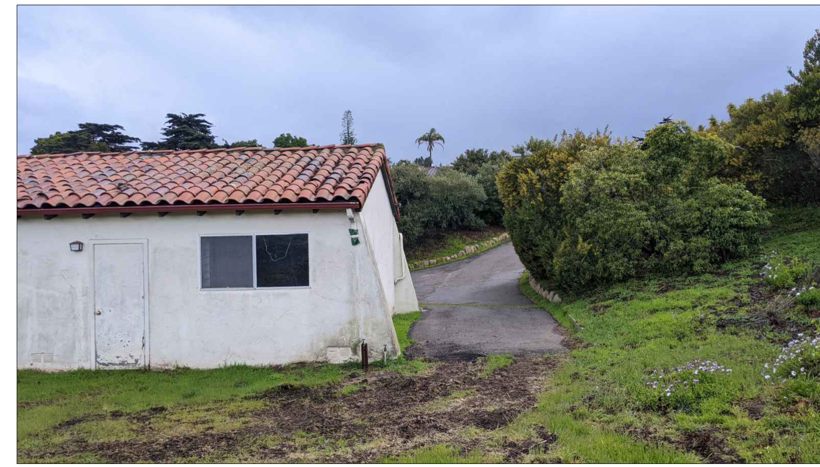
7) WEST SIDE OF EXISTING RESIDENCE LOOKING SOUTH
