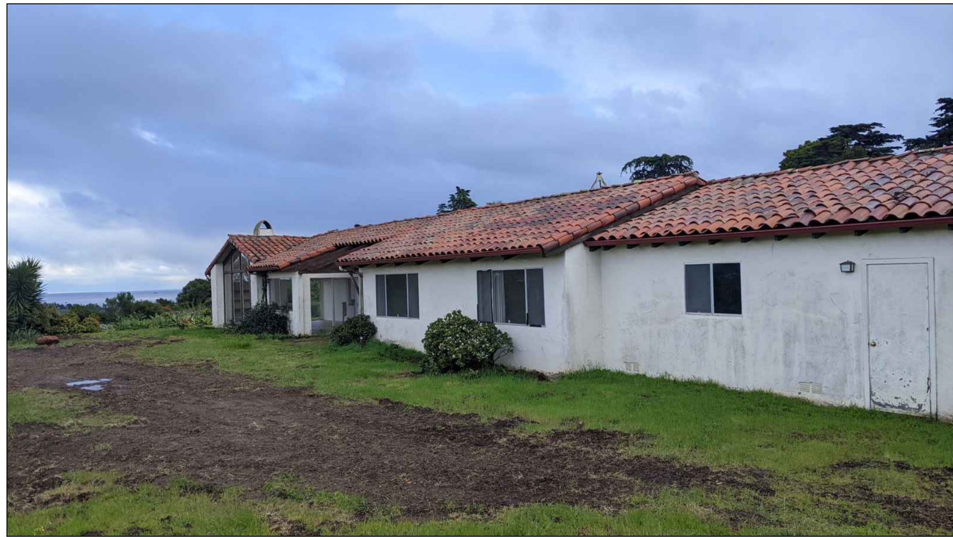
NORTH SIDE EXISTING RESIDENCE TO BE DEMOLISHED
